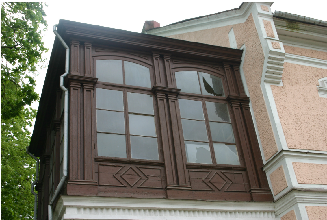
Kalna_25_62010220013001_fragments3 Verandas kopskats.
