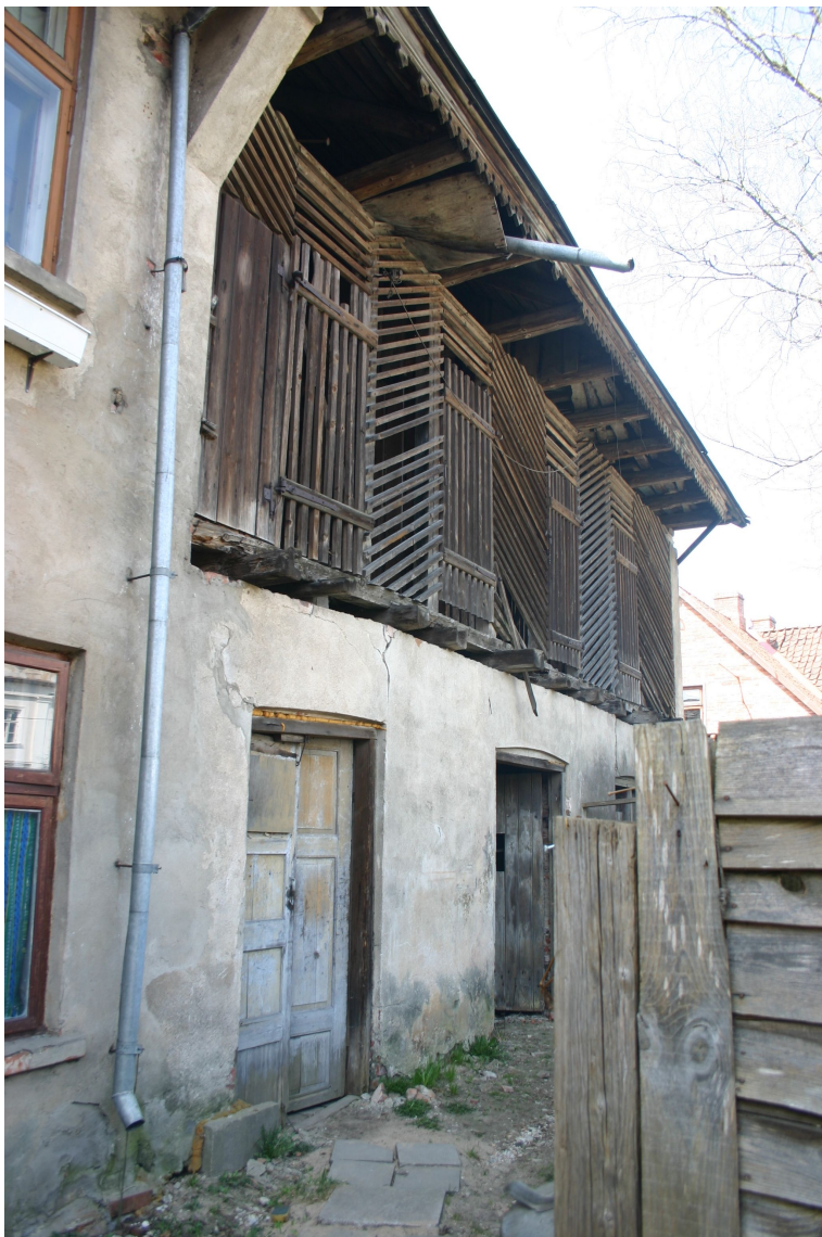
Kaljku_2_62010060013002_fasade3 Austrumu fasādes fragments.
