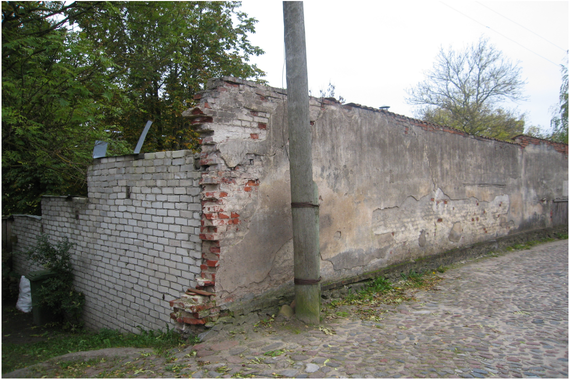
Jelgavas_12_62010220016002_003_004_fasade3 Skats uz ēkas (lit. 004) austrumu galu.
