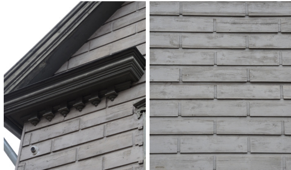
Figure 39: The façade of the building at Baznīcas Street 36 shows the typical façade design of later wooden buildings found throughout the Old town of Kuldīga, including delicately carved corner cornices
