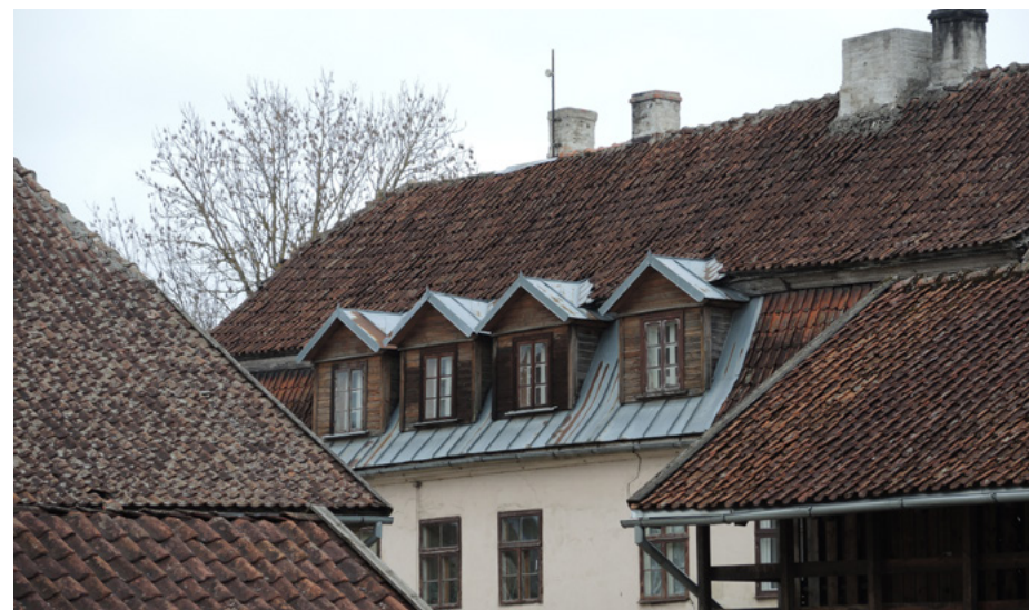
Figure 44: The roofscape of Kuldīga mirrors the 19th-century building regulations that aimed at preventing fires from spreading
