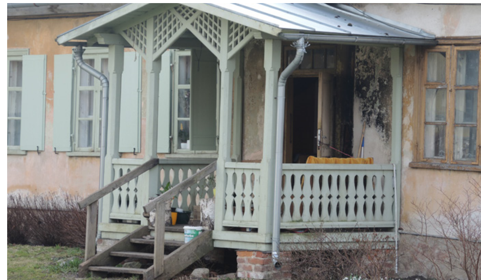
Figure 55: Porches offer a sophisticated entrance area and exist in closed and open form (here)
