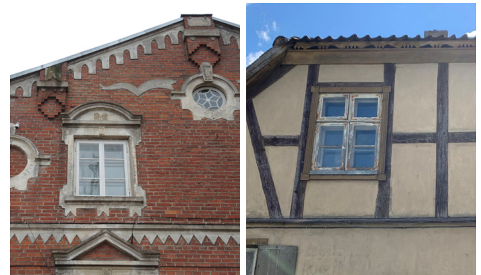
Figure 42: Mixed-method approaches (brick and plaster on the left; timber-frame on the right) show the different foreign influences and their fusion into new architectural styles
