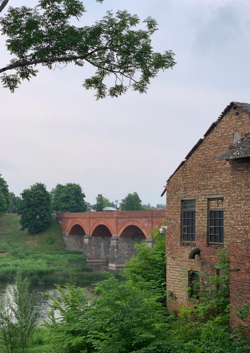
Figure 61: View towards the brick bridge from the confluence of the two rivers
