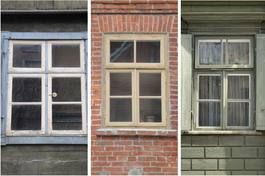
Figure 56: Examples of different front façade windows show the continuous style of the windows throughout different building periods
