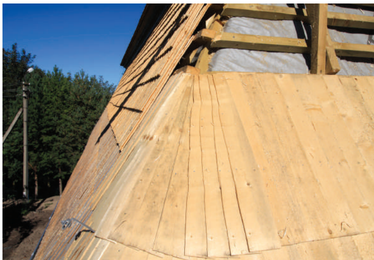
Spruce shingle roof covering 2017. (photo M. Veliulis)
