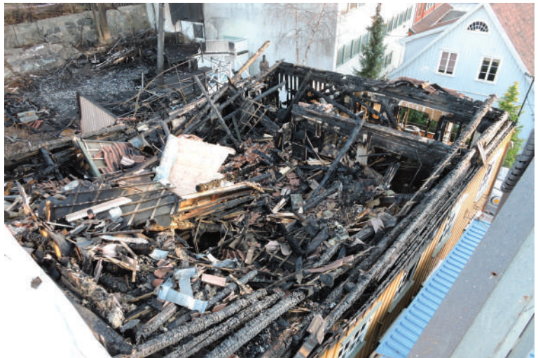
A sad view down in the fire plot, where the roof construction has burnt and fallen down on first floor. Pretty horrible chaos! The whole building was close to collapse!
