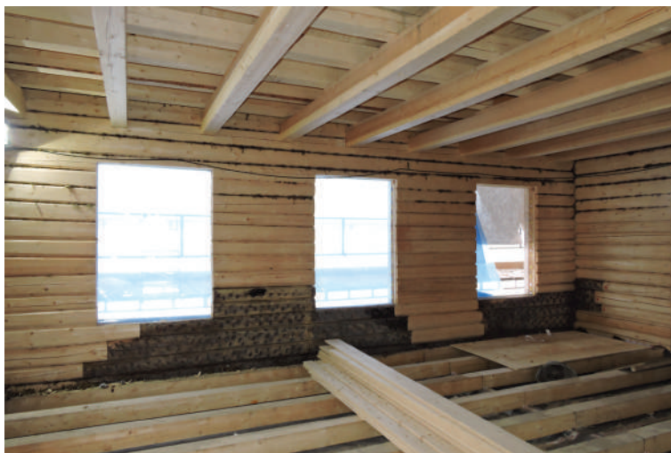
Inside the big hall in first floor, where almost all logs are new. These walls will be visible in the restaurant for several years, until the logs have been compressed and shrunk
