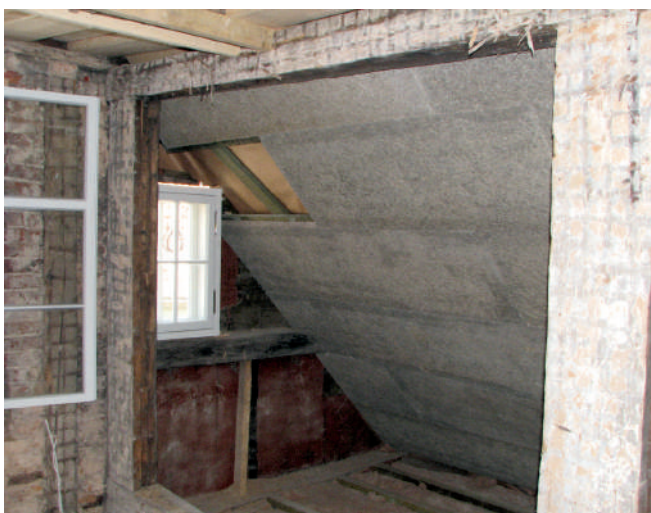
There are a steam barrier, laths and fibrolite layer placed above the wood fiber boards, afterwards the layer of the lime mortar rendering
