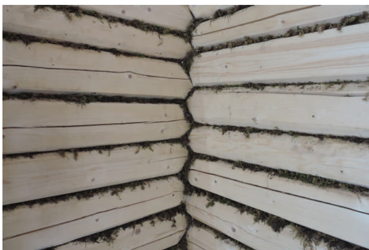
In between the logs we put wet moss ( Hylocomium splendens ) as tradition. This is absolutely the best material for this purpose, and is used all over Norway, Sweden and Latvia.
