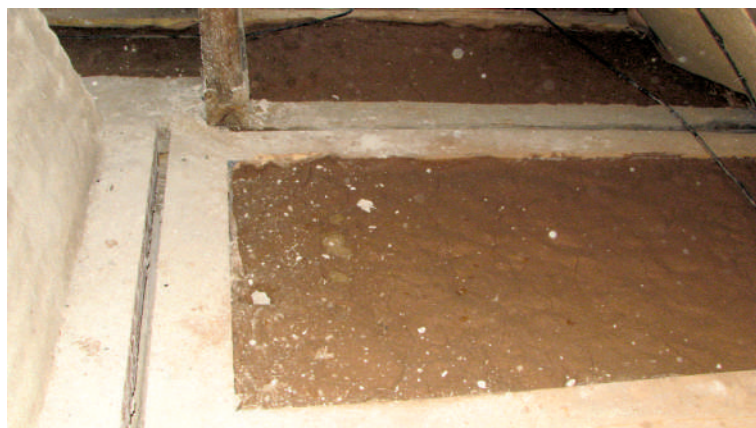
The removed and repeatedly laid clay covering
