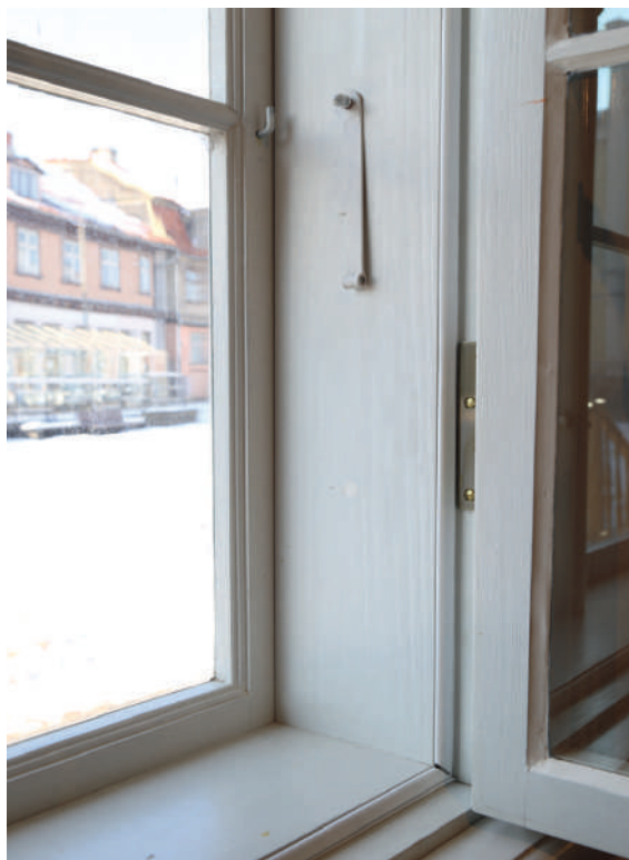
The restorable window with the applicable sealing parts in it – rubber sealing gums and the window glazing with a putty appliance in the external sashes 12
