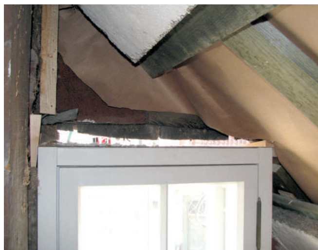
There are a steam barrier, laths and fibrolite layer placed above the wood fiber boards, afterwards the layer of the lime mortar rendering
