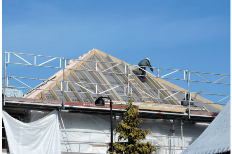
The roof insulation will be put in a rafter construction on top of the ceiling
