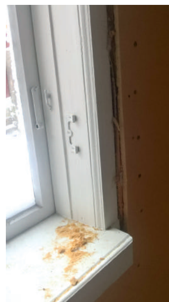
The apartment in the northern end of the building is still under construction in winter 2018. The old floor construction is in these rooms replaced with a new one. The walls are insulated with two layers of wood fiber board. Photos in 2018 Hanna Elo
