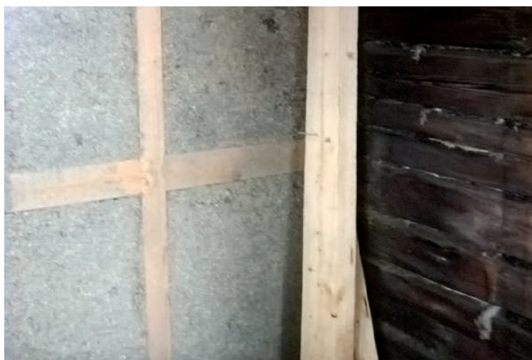
The external vestibule's framework was insulated with 150 mm of wood fiber blown directly on the frame. Photo in 2018, Hanna Elo
