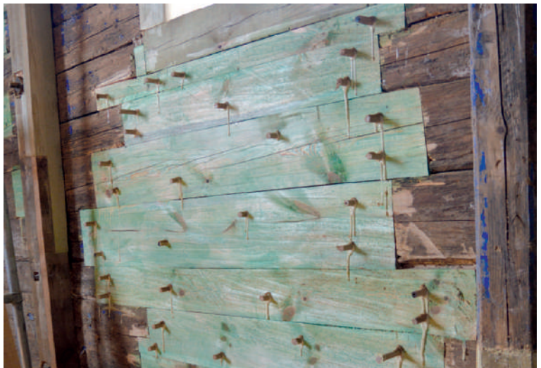
Restoration of wooden wall: implants and partial change of logs 2017 (photo M. Veliulis)
