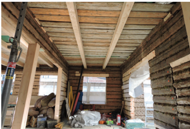
Another room in the ground floor where original ceilings is restored. The floor thickness is about 40 cm, with double crossed floor joist. Technical instalations will fit in between, and the rest will be filled up with cellulose fiber insulation
