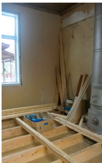
The apartment in the northern end of the building is still under construction in winter 2018. The old floor construction is in these rooms replaced with a new one. The walls are insulated with two layers of wood fiber board. Photos in 2018 Hanna Elo
