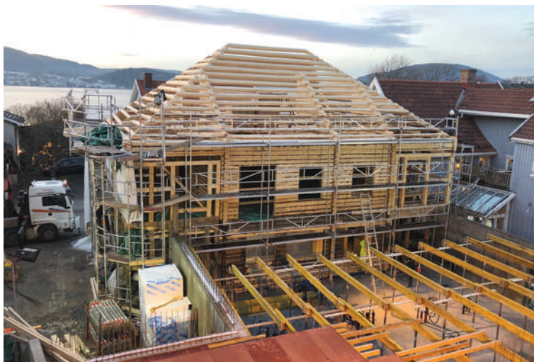
On the 5th. of December 2017 the whole building was back in town, risen up from the ash! The roof construction contains of 850 meters of round logs. In front is the roof of the new kitchen under construction. The kitchen will be moved outside the old building
