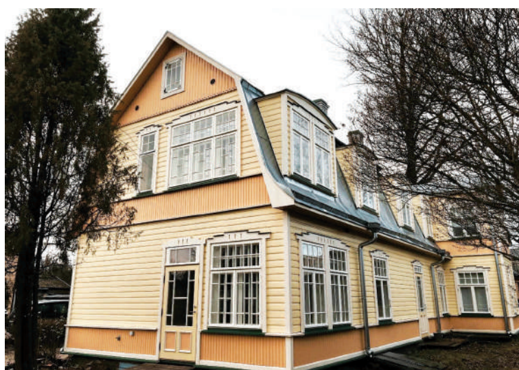
House after renovation. Photo: J.Laineste
