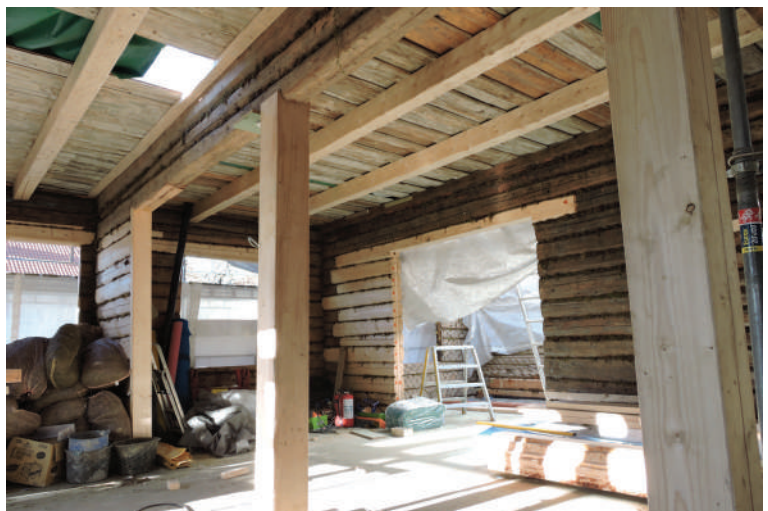
Inside to rooms in ground floor, where we see original ceilings and log walls. The ceiling joists and part of the walls had to be made new
