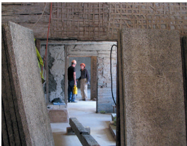
And their dismantled materials which were used in 1973 for reconstruction, including the fibrolite boards
