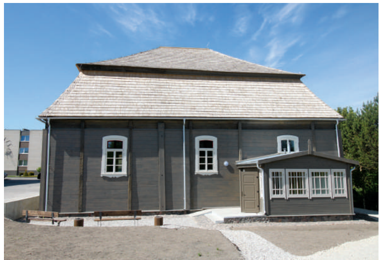
The synagogue after restoration 2017.
