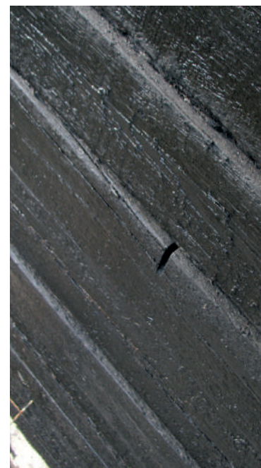
The restored walls – caulked, afterwards pitched wooden log-house walls
